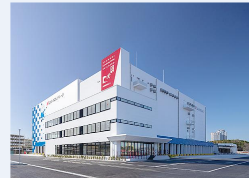
Nagoya Minato DC Solar panels scheduled for installation in March 2023
