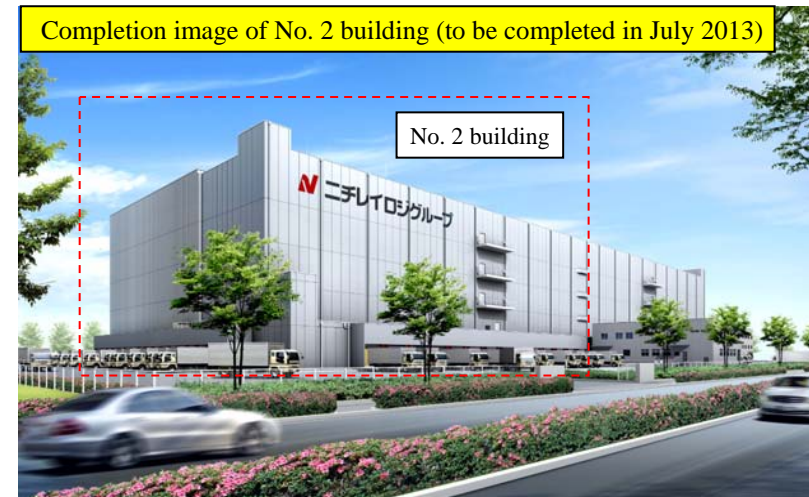
Higashi-Ogishima DC (No. 1 and No. 2 buildings)
