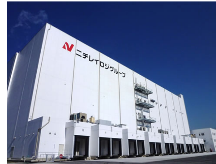
Main facilities of Higashi-Ogishima DC
