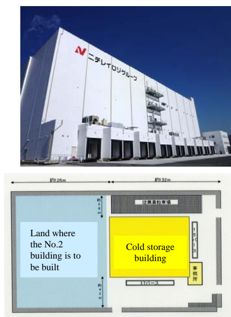
Main facilities of Higashi-Ogishima DC
