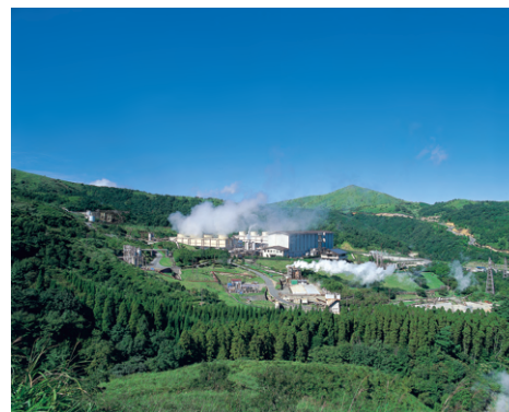
Geothermal Power Plant (Kyuden Mirai Energy Co., Hachobaru Power Plant)
