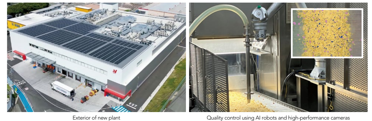
Exterior of new plant
