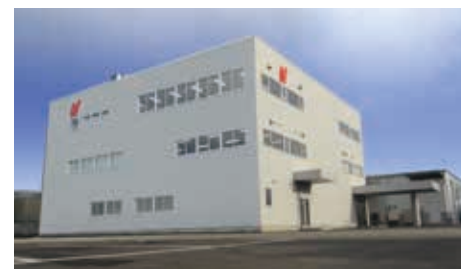
Overview of Funabashi No. 2 Plant (Nichirei Foods) Total investment: Approx. ¥6.2 billion (Land and construction, etc.)
