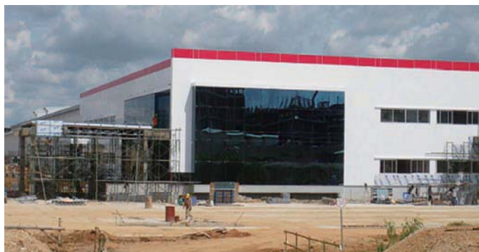
GFPT Nichirei, under construction
